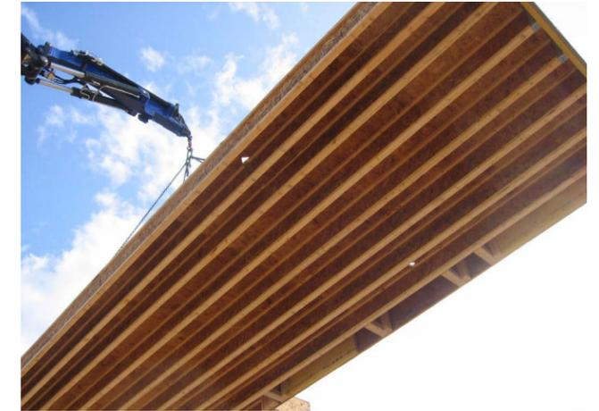
Crane lifting Home Technology's floor panel into place.
