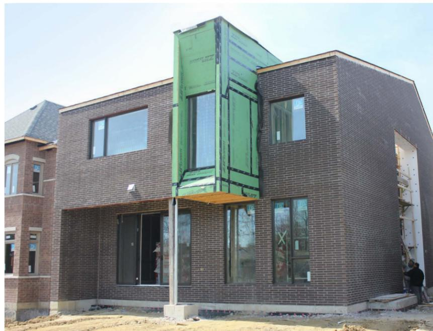
Rear exterior elevation stucco application being installed.
