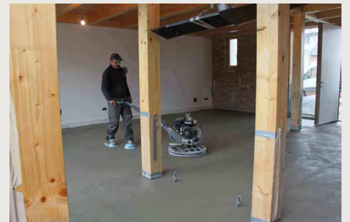
Concrete finishing
