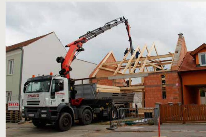
Erecting of roof truss
