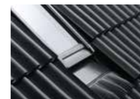
Featured: EDJ recessed tile installation.
